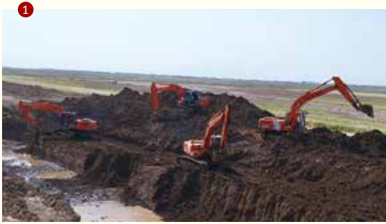
① 曝气池土方开挖 Aeration tank excavation
