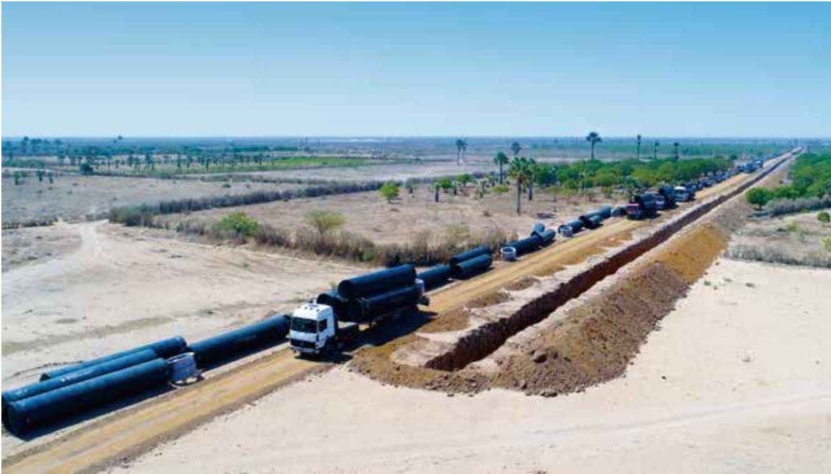
塞内加尔KMS3-LOT6项目：55公里球墨铸铁管线供货和铺设 Supply and Laying of 55 KM Ductile Iron Pipes of KMS3-Lot 6 Project in Senegal
