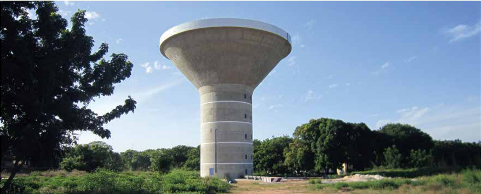
塞内加尔ZIGUINCHOR城市加压输水管道及3200方水塔工程 Elevated water tower of 3200 m3 and water supply pipe lines of the city of Ziguinchor, Senegal
