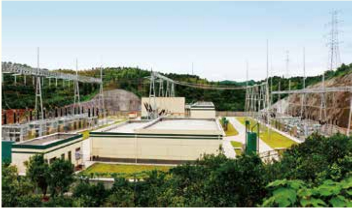
抚州七里岗220KV变电站工程 配套220KV输电线路工程 (电站规模150MVA, 输电线长度22km) 220KV Substation Project in the town of Qiligang, Fuzhou City and 220KV Power Transmission Line, China (Capacity of substation: 150 MVA, length of transmission line: 22km)
